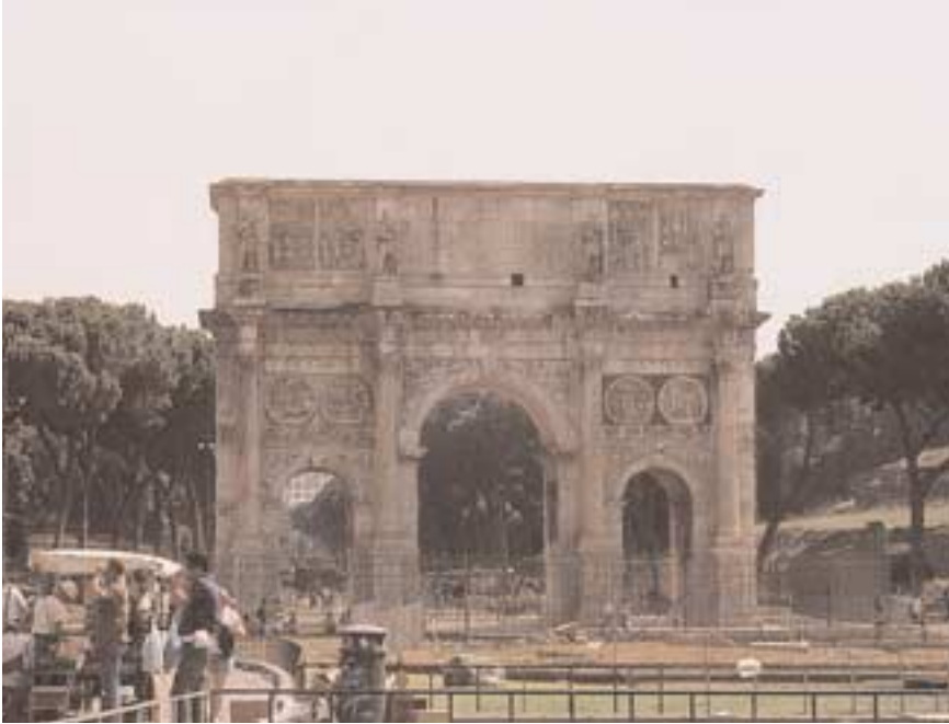
The Arch of Constantine in Rome (built in 4th century) is an example where recycled marble from former Roman constructions was used. It is an ideal example demonstrating that stone has long been recycled.
