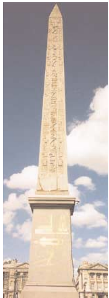
The Obelisk in the Place de La Concorde was manufactured from granite in Ancient Egypt in about 1300BC. It exemplifies the durability of stone as well as stone recycling.
