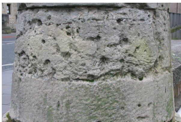
Fig. 5a Differential weathering of limestones that have local patches of micrite with high microporosity in them. 5a, micrite-rich burrows in (probable) Headington Stone weathering out to give cavernous texture. 5b, micrite-rich laminae in Milton Stone.
