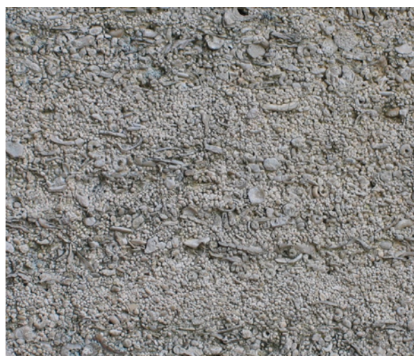
Fig. 1. Detail of excellently preserved Barnack Stone mediaeval ashlar in Bury St. Edmunds, showing minimal weathering decay over several centuries.
