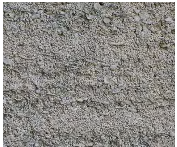
Fig. 1. Detail of excellently preserved Barnack Stone mediaeval ashlar in Bury St. Edmunds, showing minimal weathering decay over several centuries.
