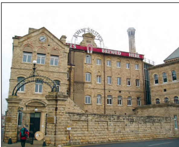
Figure 8 Smaws Quarry has long been owned by the Smith family, Tadcaster brewers since 1758. The town's chief landmark and triumphal monument to Smaws stone is their massive rock-faced brewery.
